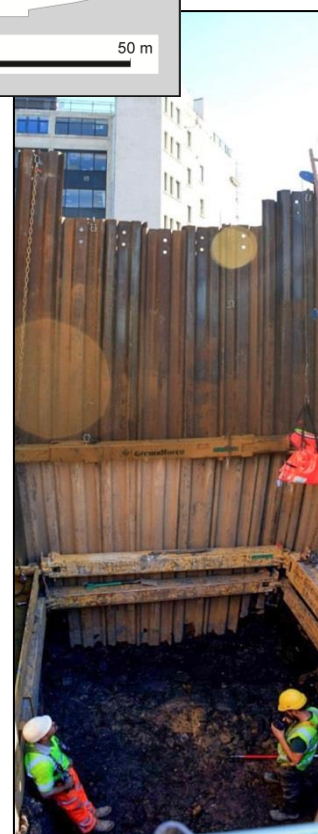
Figure 7 Shoring of Trench 10
