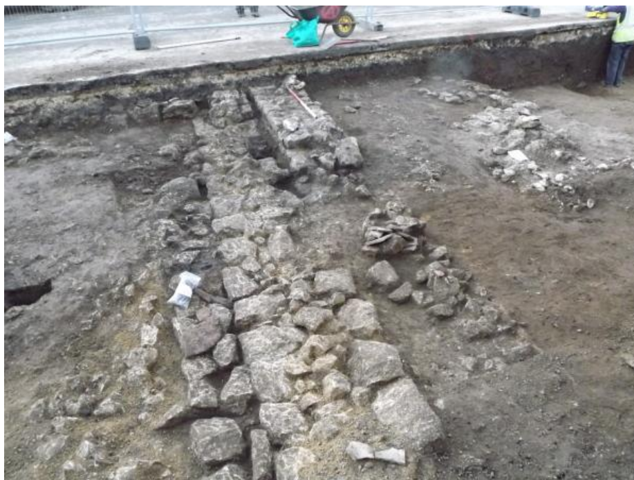
Figure 3 Remains of two substantial 'warehouse like' building located cable end to road (Scale 1m, looking west)
