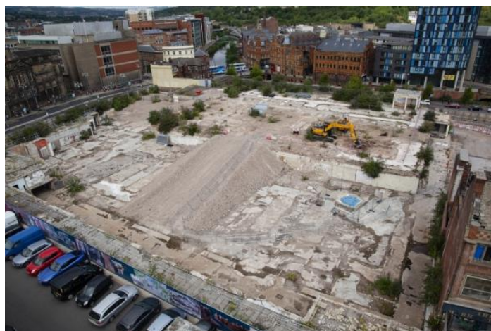
Figure 5 Birdseye view showing different levels, concrete and remaining structures of the Castle Markets
