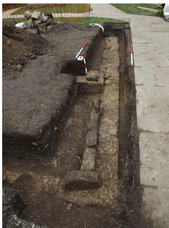
Figure 1 Foundations of the western wall of the 1755 cottage, looking south-east scales 0.5&1m © J Buglass
