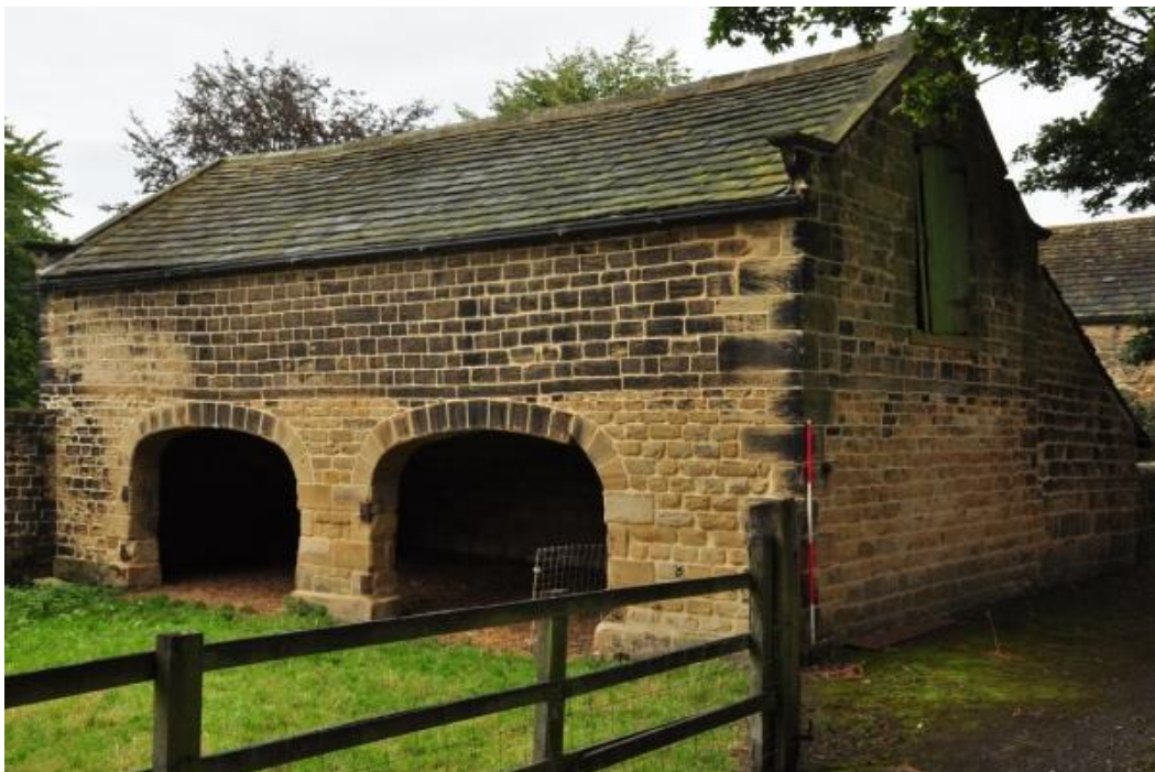
Figure 4 Cart-shed and granary, Heath Hall Farm, Wakefield. Copyright Stephen Haigh. https://doi.org/10.5284/1057510
